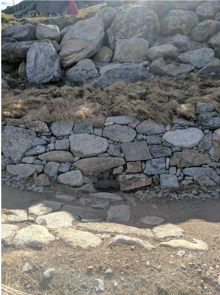
Figure 17: Example of a drain dip, rock hardened on the All-Mountain Trail
