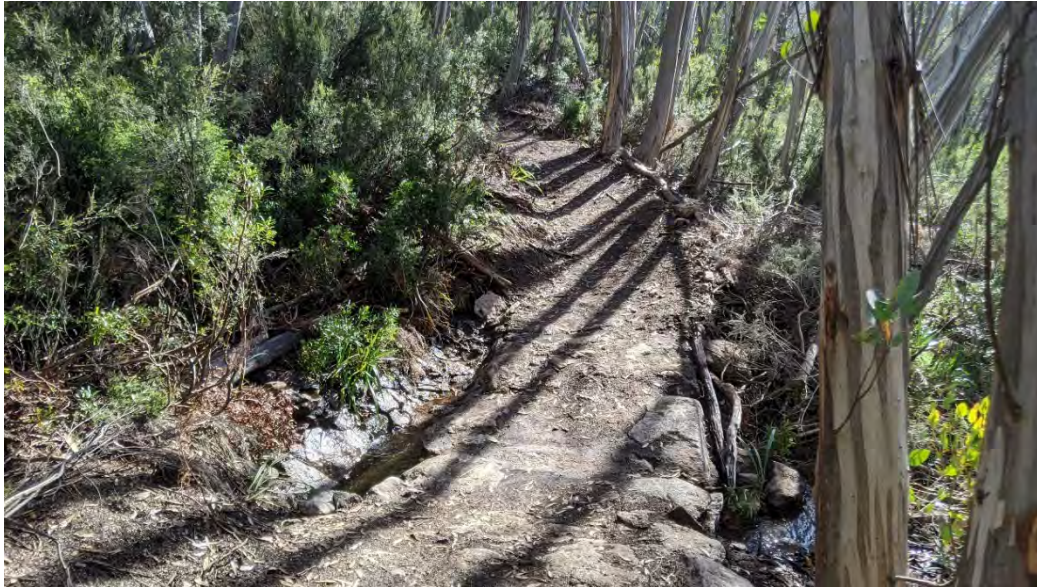
Figure 18: Example of rock armouring on the Sidewinder Trail
